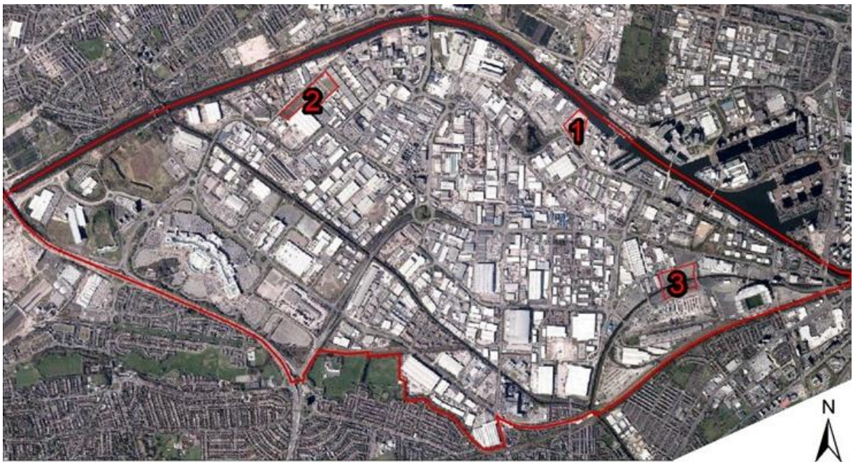
Figure 25: Potential Site for Energy from waste facility
